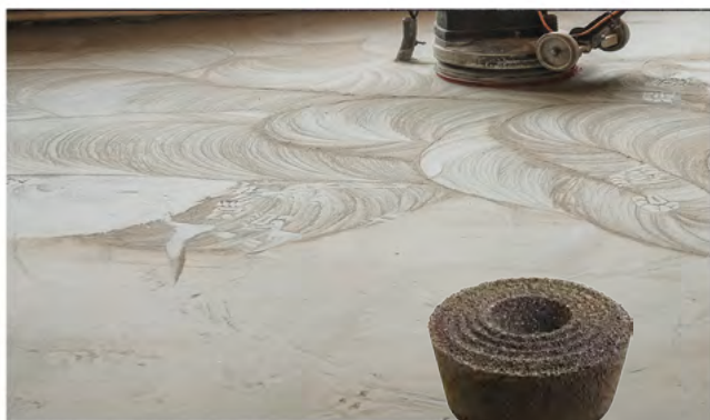
Alfa Mola Cylinder silicon carbide designed for leveling concrete substrates and eliminating creases.
